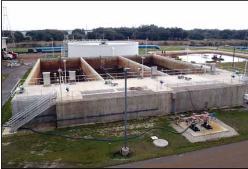
Figure 4. Three new backwash clarifiers remove solids before discharging to recycle basin.
