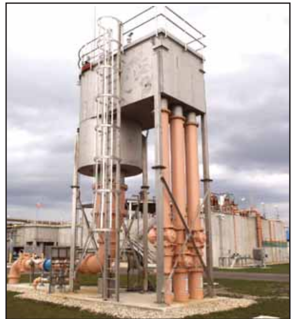
Figure 5. Gravity thickener influent mix chamber enhances settleability of solids in the gravity thickeners.
