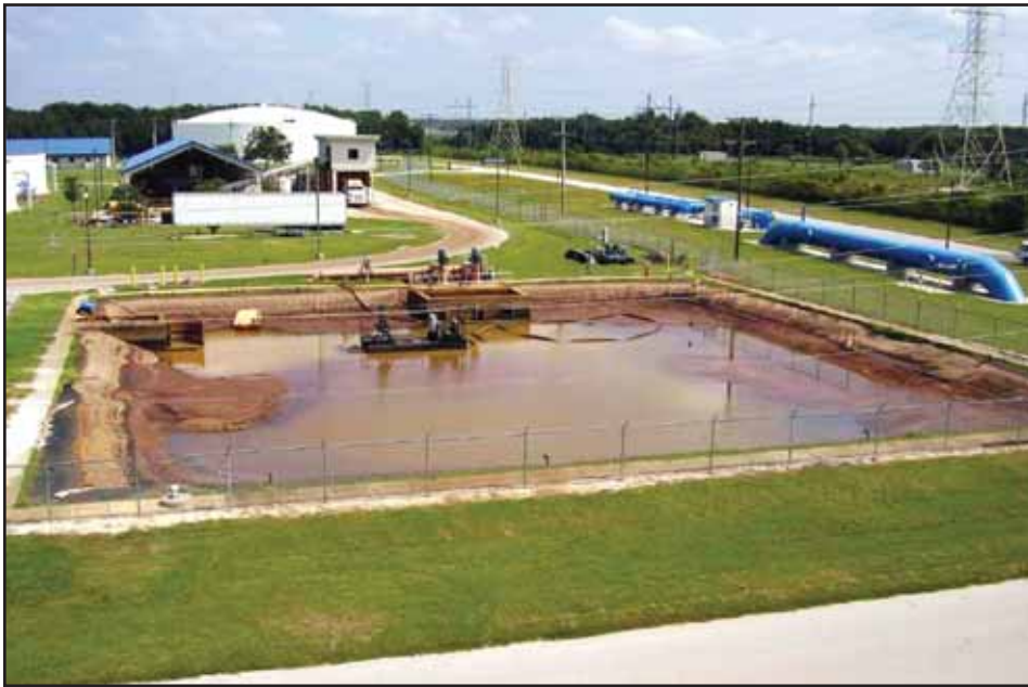
Figure 2. Recycle basin nearly half full with solids before improvements.
