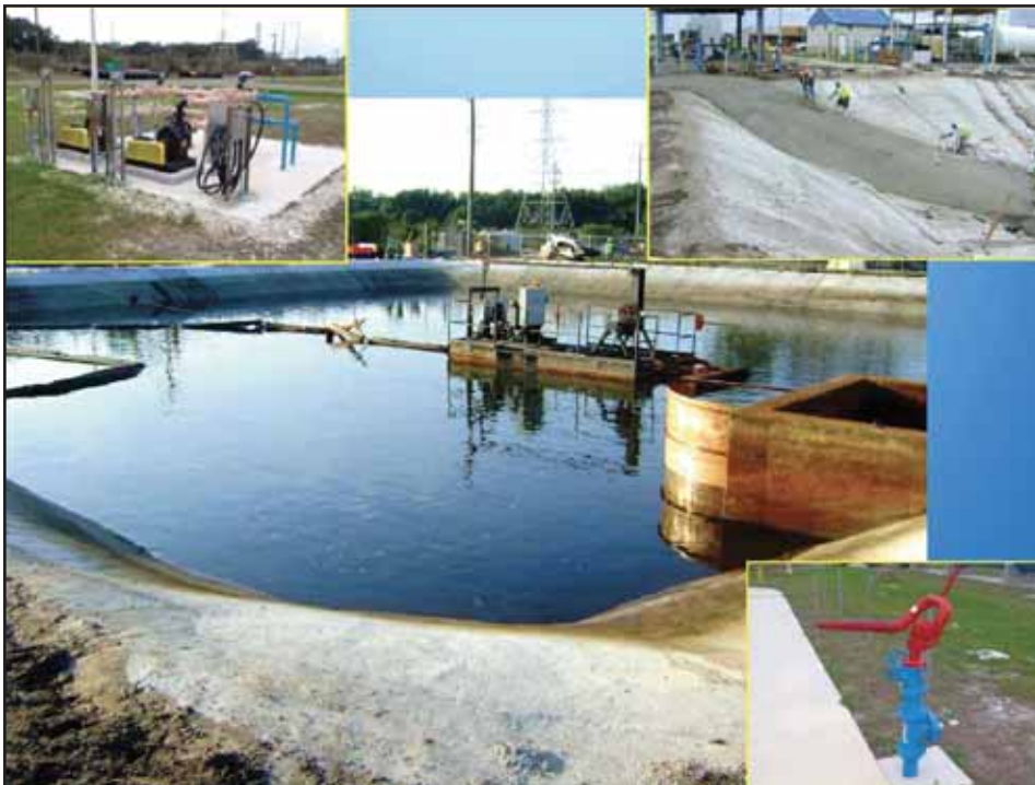
Figure 6. Improvements to recycle basin provide better solids removal and minimize accumulation.
