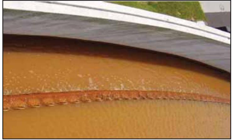
Figure 8. Intermittent side stream flows and poor polymer dosing/mixing led to high solids carryover in the gravity thickeners.
